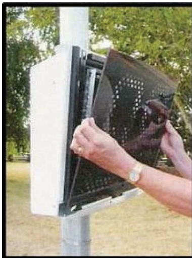
Tilt window forward & lift to remove.
