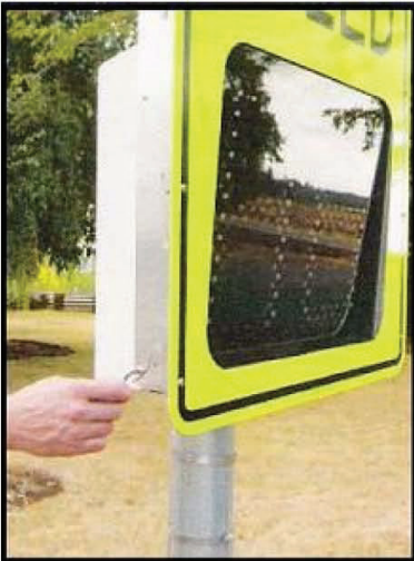
Remove the two fasteners, one on each side.
