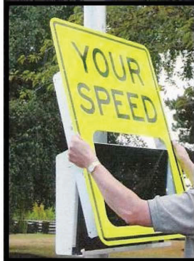
Tilt sign to rear and lift to remove.
