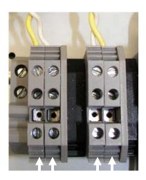
The Flasher System can be turned **OFF** by lifting the 4 Amp fuse holder.
