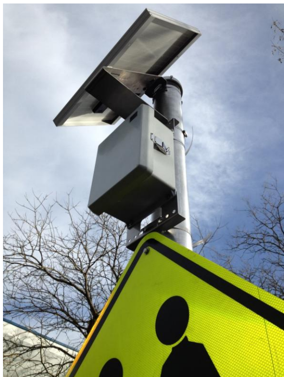
Figure 4-0-2: AC and Solar pole mount configurations
