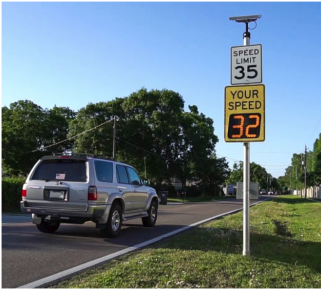
Radar speed feedback sign installed on same post as Speed Limit sign
