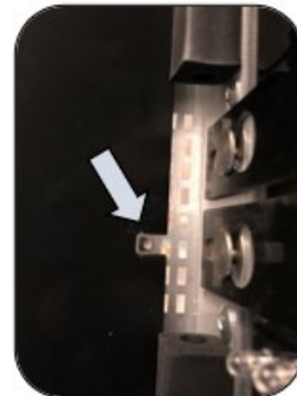
Take note of window alignment stud for re-installation
