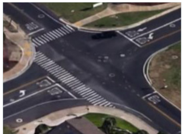
Four-way stop intersection before roundabout installation
