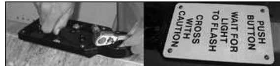
Figure 21: Push-button plate and sign (right)
