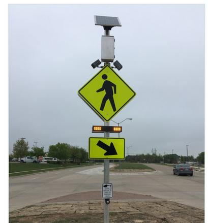
The church's new crosswalk includes advance warnings on the approach, as well as passive detection on three poles at the crossing.
